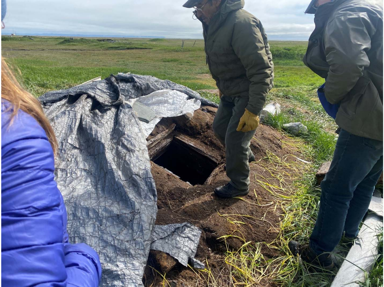
Figure 4. A Point Hope elder Henry Koonook, showing the field team his active ice cellar (Traditional Siglauq), which is accessed through the vertical shaft over the top of the subterranean structure. The Field Team installed dual channel temperature sensors in four ice cellars at Point Hope to collect data that can inform how climate change is impacting the community. Photo taken by Katie Dunn on 22 July 2021. IMG_0012.jpg.
